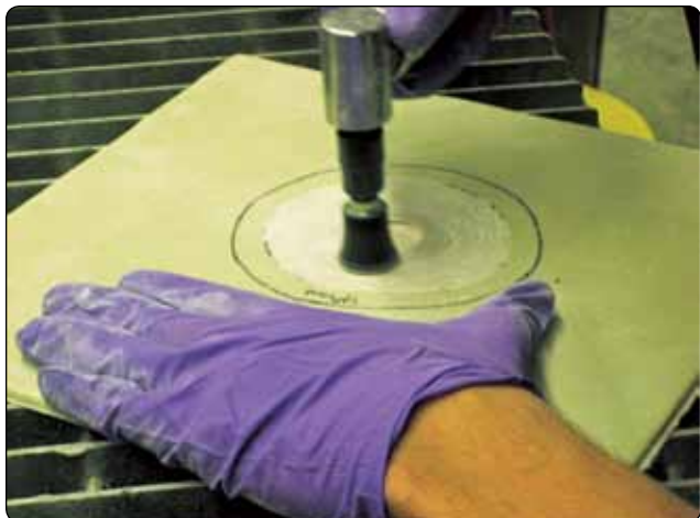
Figure 7-58. Taper sanding of repair area.
